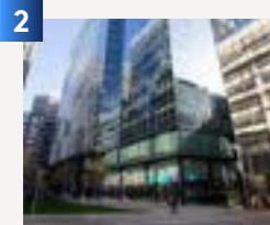
2 ONE BRAHAM STREET Union 343,000 sq ft offices and retail Completed - 2020
